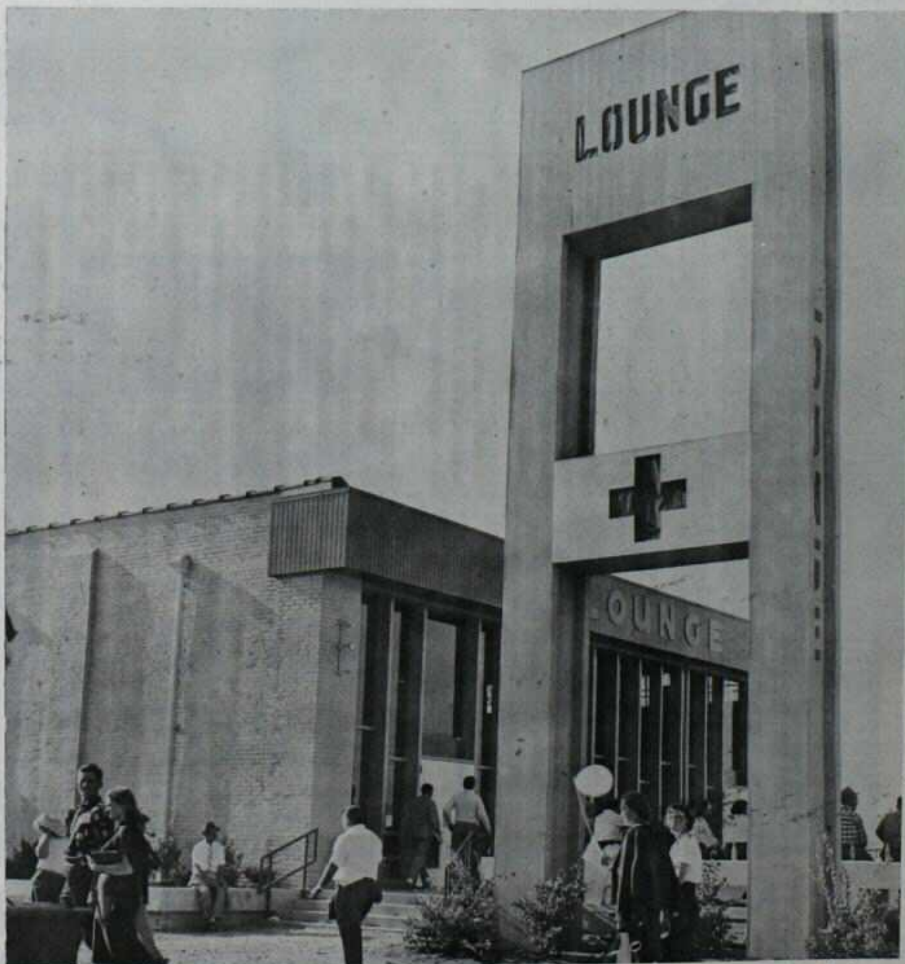
A typical Doc Dorton touch, a large, attractive and inexpensive sign identifies the combined lounge and first aid building at the North Carolina State Fair, Raleigh. The sign is made of plywood, placed over 40-foot high light poles.
