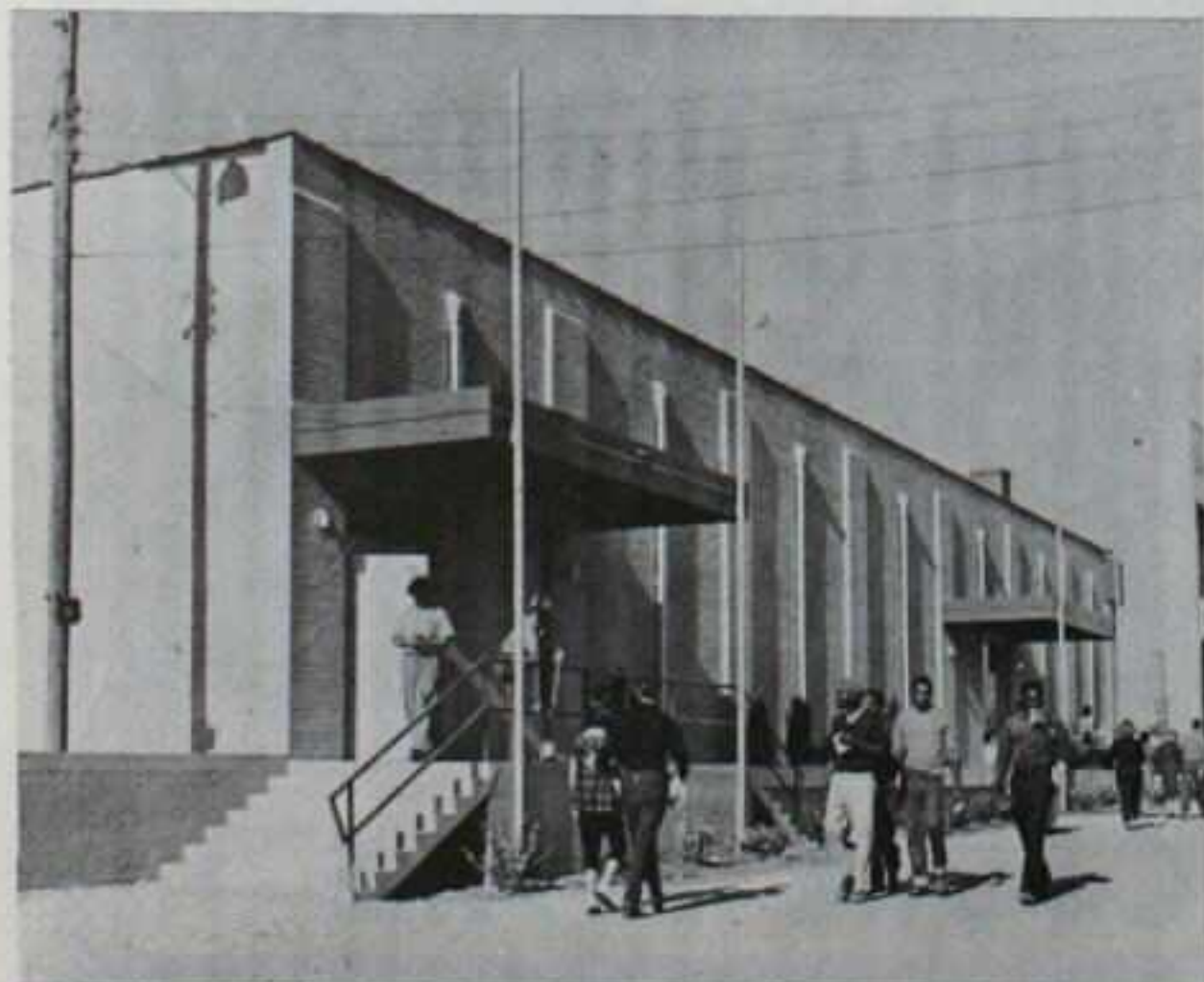
Rest rooms for men and women with outside entrances add to the utility of the new combined lounge-first aid building.
