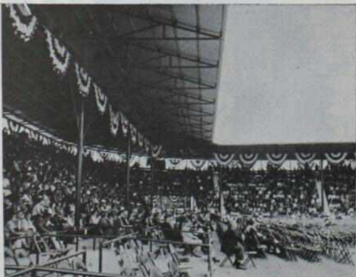
The alertness and resourcefulness of Clyde Byrd, manager of the Arkansas Livestock Show, Little Rock, gave that up-and-coming event a new grandstand in '58 at low cost. Learning that the Texarkana baseball plant was to be abandoned, Byrd purchased its stand, had it knocked down, moved to Little Rock, and re-assembled. The result is shown above.
