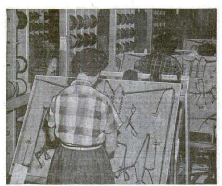
The complex wiring of the modern juke box gets its start with this ingenious new arrangement of spools and harness boards. Here deft operators tie hundreds of feet of vari-colored wires into compact networks that transmit electrical impulse with unerring accuracy.
