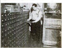
SMALL PARTS BIN OFFERS convenient stocking of miscellaneous unifs vital to continuous trouble-free operation, Individual drawers, numbered and carrying labels describing contents, permit easy checks on spare parts backlog plus enabling operator to find given items in the least possible time.
