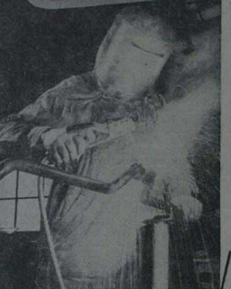
Extra strength where it's needed the most. Crank-rods and other vital parts are welded to give long, trouble-free performance.
