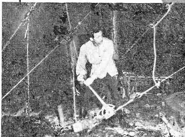
Castle is shown tightening his bounding wire with a 1½ ton capacity, Model F.G. Safety-Pull Ratchet Lever Hoist. Other Coffing Hoist Equipment shown at left is Midget Puller, 500 lb. cap., weight 6½ lbs.; center, Safety-Pull Ratchet Lever Hoist, ¾ ton cap., weight 14 lbs.
