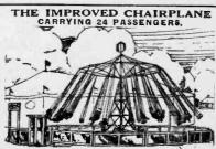
The Chairplane can be had in two heights with 18 ft. and 22 ft. towers, making the entire heights 26 ft. and 80 ft. The 18-ft. tower ride has shorter sweeps, consequently can be operated on smaller space and under most trees and overhead wires. Newly arched exit and entrance signs and improved ticket booth have been added at no extra cost. Please write for prices and description. description. SMITH & SMITH, Springville, Erle Co., N. Y.
