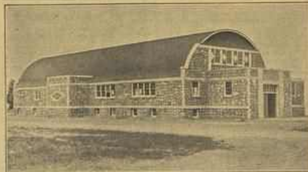
FESTIVAL HALL, recently completed on Wells County Free Fairgrounds, Ferdinand, N. D., was designed by and built under supervision of Secretary Edward W. Vancura. It is 44 by 134 feet, two stories, of cut rock found in the county, and was constructed by WPA labor. Building is air conditioned, basement floor is for industrial and farm exhibits, and an auditorium is on the main floor.
