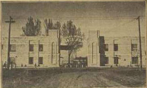
ADMINISTRATION BUILDINGS AND ENTRANCE to Eastern Idaho State Fair, Blackfoot, shown here, have been erected at a cost of $25,000. Twelve counties contribute toward support of the annual. About $90,000 in improvements have been made in the past three years, reported Secretary-Manager Eric Sundquist. A new grandstand has been built at a cost of $23,000, a large commercial building cost $26,000, other buildings have been remodeled, and there has been much landscaping.
