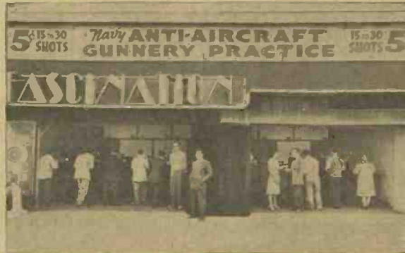
A BATTERY OF KENEY ANTI-AIRCRAFT GUNS has made the above Ocean Park, Santa Monica, Calif., location one of the West Coast's most popular, reports Barney Fishman (center foreground), who made the installation.
