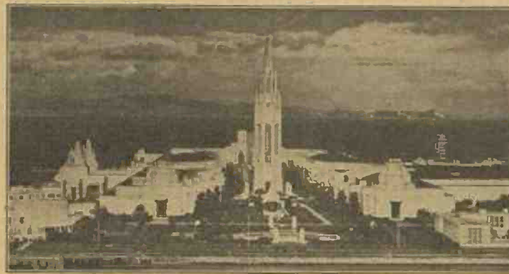
LOOKING DOWN FROM NEAR-BY YERBA BUENA ISLAND, this sectional photograph of the site of Golden Gate International Exposition, San Francisco, shows the Elephant Towers at the main entrance (left) and the 400-foot Tower of the Sun (center). In the foreground is the sunken garden with Yerba Buena women's clubhouse at the right. Atop the central tower is the Golden Phoenix.
