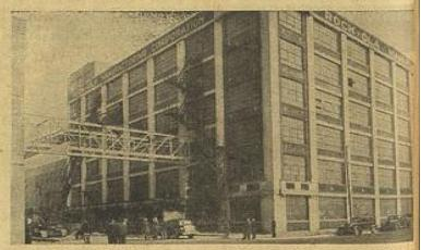
DERRICK AND STEEL are symbolic of progress. Above is a scene taken of the Rock-Ole factory, Chicago. Workmen are constructing an aerialway to had the main building to an auxiliary building across the street.
