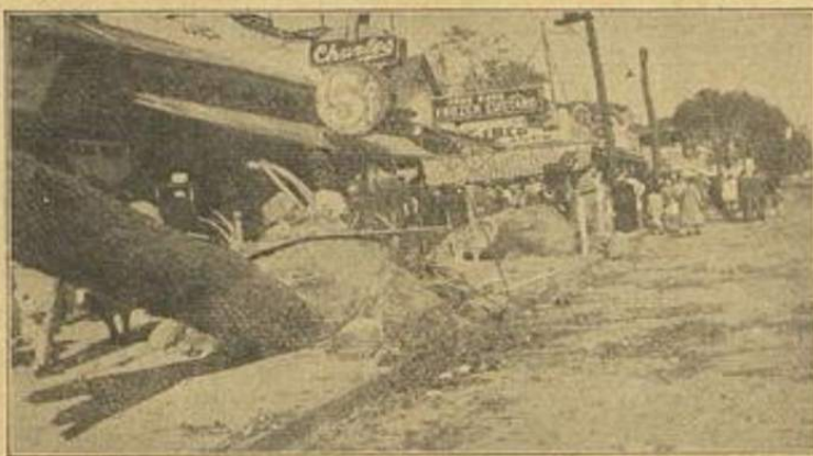
CROWDS VISITED SAVIN ROCK PARK, near New Haven, Conn., after the hurricane of September 21 and saw giant trees felled and clearance work being started immediately to rebuild the resort. View was taken on Beach street, where most damage was done, by Andrew T. Colarolpe.
