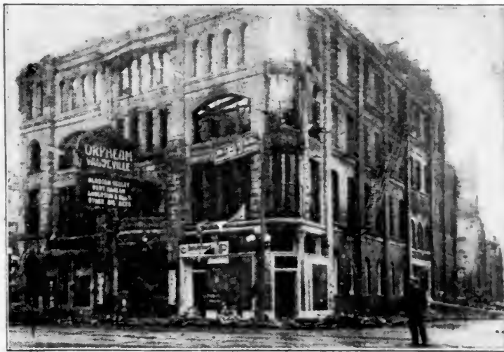
What was left of the Orpheum Theater, formerly the Grand Opera House, at Memphis, Tenn., after it was gutted by fire Thursday night, October 18.
