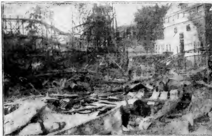
Herewith is pictured a part of the $125,000 damage done by fire to Chester Park, Cincinnati, July 18.
