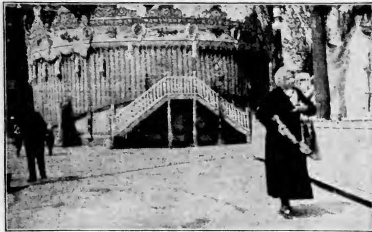
Set of gondolas taken before they opened. Notice all the flaming arc lights.
