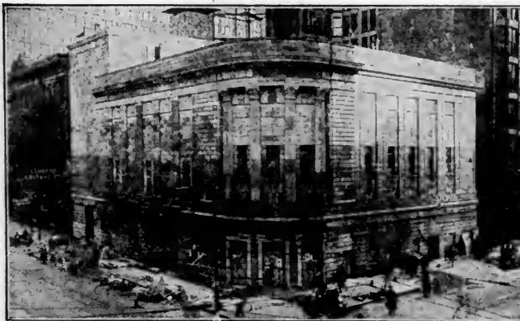
The Apollo, which is A. H. Woods' new Chicago theater, is nearing completion. It is a magnificent house and was designed by Hotelard & Roche, architects. —Photo by Chicago Architectural Photographing Co.
