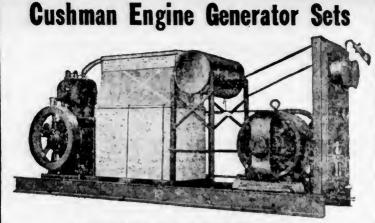
20-H. P. POWER PLANT, WITH STANDARD TANK COOLER Automobile radiator equipment with cooling fan may be had instead of tank cooltr. Special switchboards obtainable for individual requirements. Adapted for all annusement houses and devices requiring electric power or light, from the smallest moving picture theater to the largest road show
