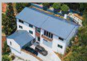
The crew's home in the Hollywood Hills.
