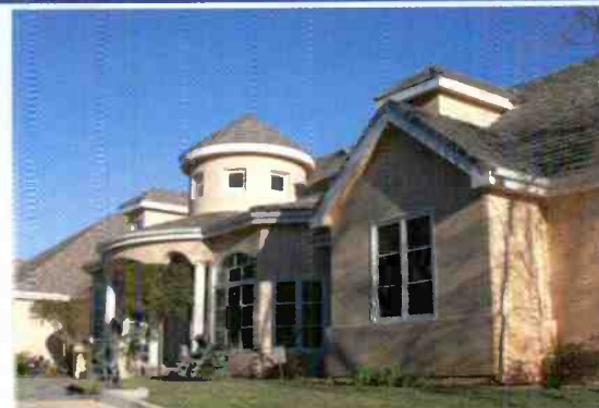
North Ranch • Westlake Village Southern California
