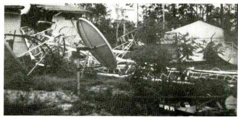
An F-15 fighter jet hit a guy vire Friday (5/19) and demolished the 1464-foot tower, located near Clarksville, FL, shared by WPAP/Panama City and two TV stations. The tower's crash also crushed WPAP's service building, but no one on the ground or in the jet was injured. Based on the evidence pictured above and last week's Page 1 transmitter carnage, it's been a tough couple of weeks for towers.
