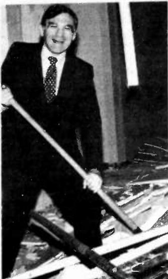
CLEANING HOUSE — Looks as if ABC Radio Enterprises Programming VP Rick Sklar is doing his fair share as construction begins on the ABC Superadio satellite programming center , located at 1700 Broadway in New York. Upon completion, plans call for the July '82 debut of an A/C format originating from the center.
