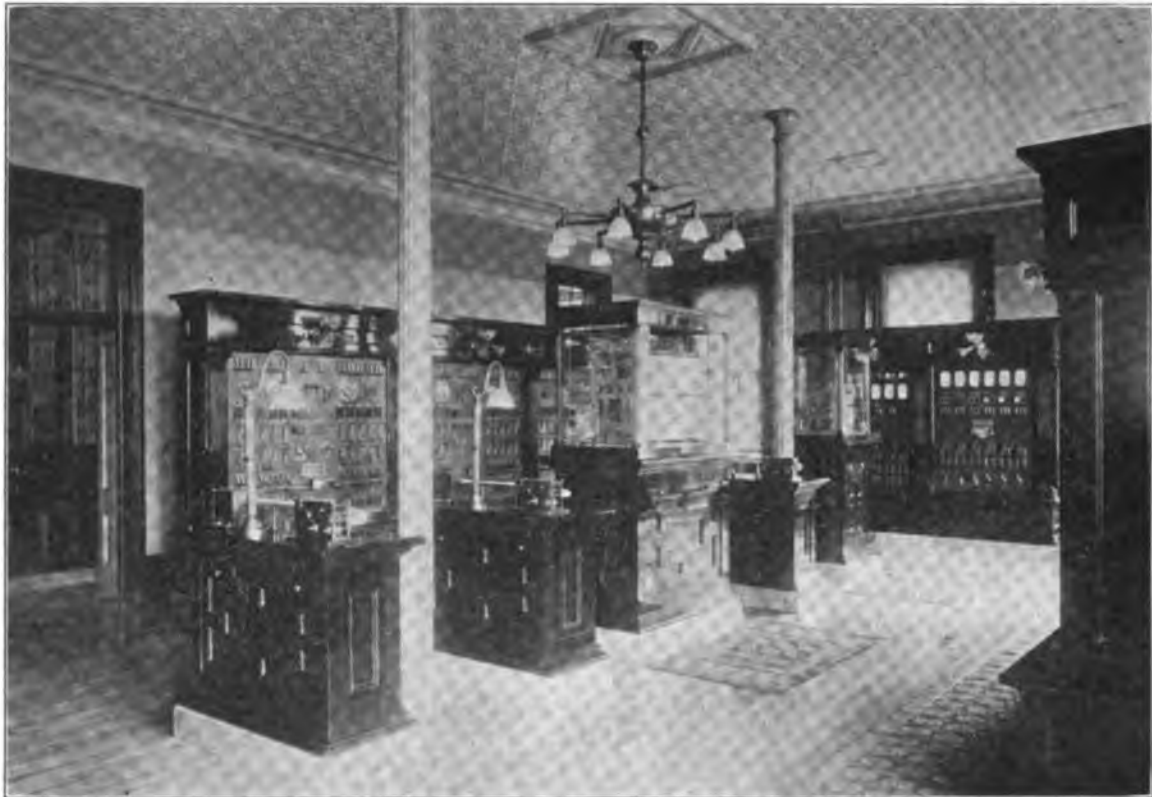
ALBANY FIRE ALARM INSTALLATION.
