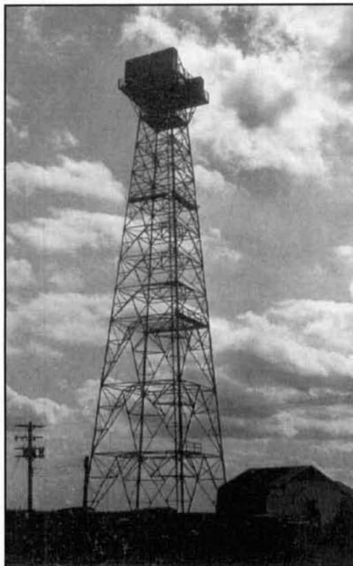
Photo H. One of the first microwave antennas and relay towers used across the nation. The antenna towers were capable of receiving and relaying messages over several hundred channels and television signals. (Courtesy of Bell Telephone Laboratories)
