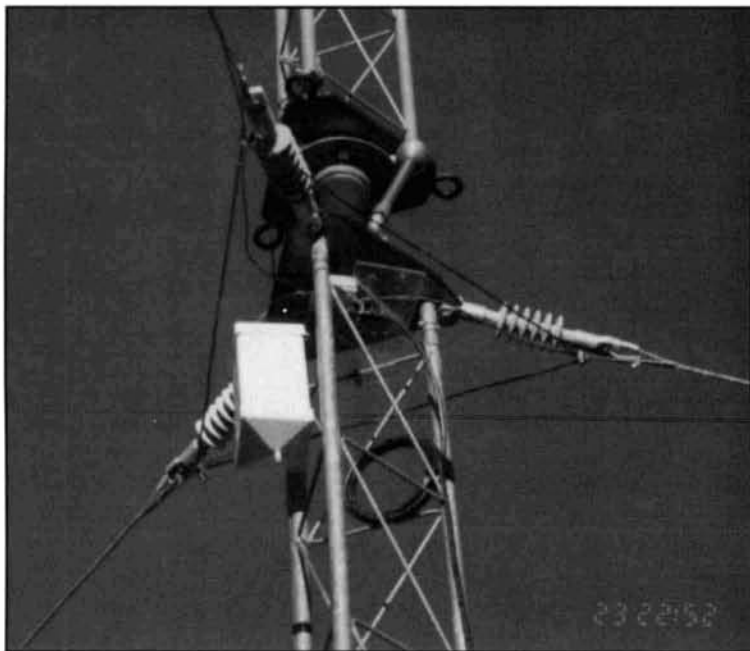
Photo B. Radial feedpoint connection.
