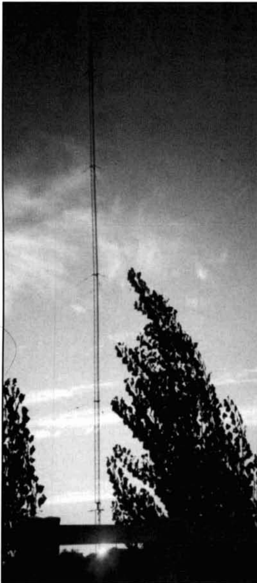
Photo A. 160-meter vertical with three elevated radials.
