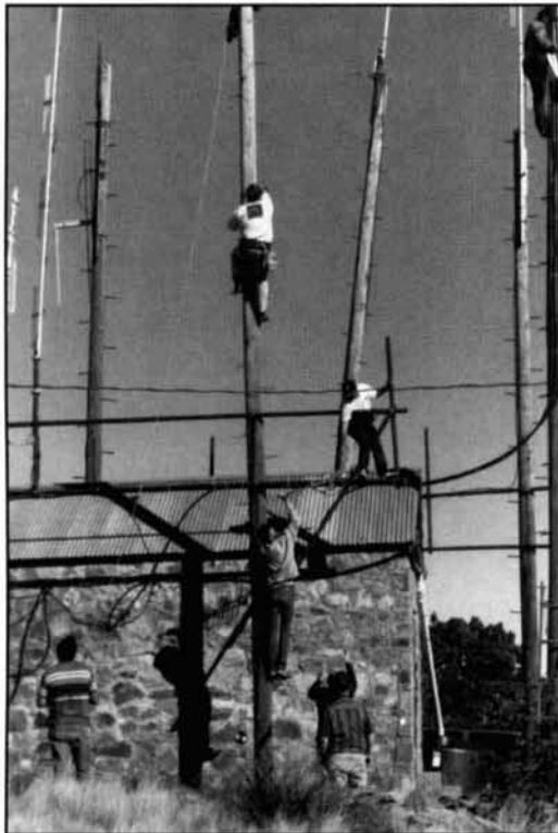
Photo A. Remounting antennas. Guests from Houston, Ft. Stockton, El Paso, and Monahans, Texas, assist members of Intertec, Inc., in relocating antennas at the Mt. McElroy site in the Davis Mountains of west Texas, 6,693 feet, AMSL. This station overlooks Pecos and Ft. Stockton, as well as the junction of I-10 and I-20, en route from Houston and Dallas to Los Angeles. One of the telephone poles had fractured and feedline on one of the link antenna coax runs was soaking wet and corroded. We replaced all hard line runs and connectors. We secured each to the poles with #14 insulated solid copper wire, taped all connectors with Scotch 23™, then thoroughly varnished each taped connection with Scotchkote™.
