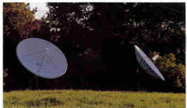
At TV 43, primary programming is received on a fixed Microdyne antenna. The VistaLink antenna rotates to receive programming from other satellites.
