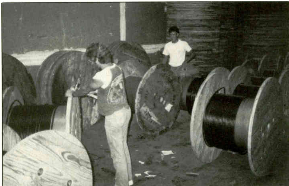
Organized and systematic reel disassembly and cable retrieval.
