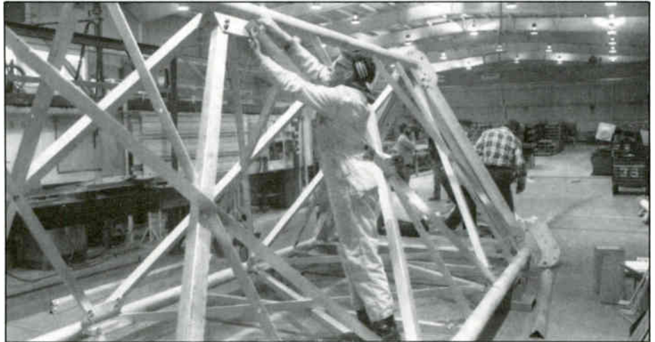
A construction team assembles the tower.
