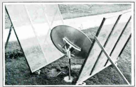
System of reflecting screens to protect a TVRO located midway between two AT&T towers emitting a total of 12 carriers. All 24 channels were initially blank. Screens plus IF traps created acceptable pictures. Cost of screens: approximately \$250 for labor and materials.
