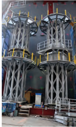
The different tower sections during construction
