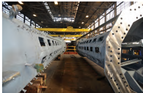
The massive tower sections layed down in the field yard.
