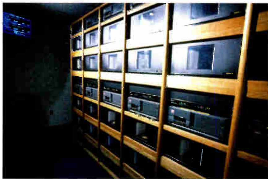
A special room was built at Greater Media's Morrissey Blvd. facility in Boston to showcase the CD jukebox array. Custom furniture was made to house the players. The TV in the upper left showed what was playing on any of the five stations.
