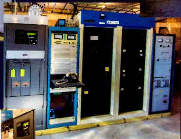
Transmitters and phasor for WHMH(AM).
