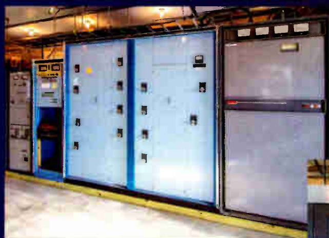
WVAL transmitters and phasor are shown.
