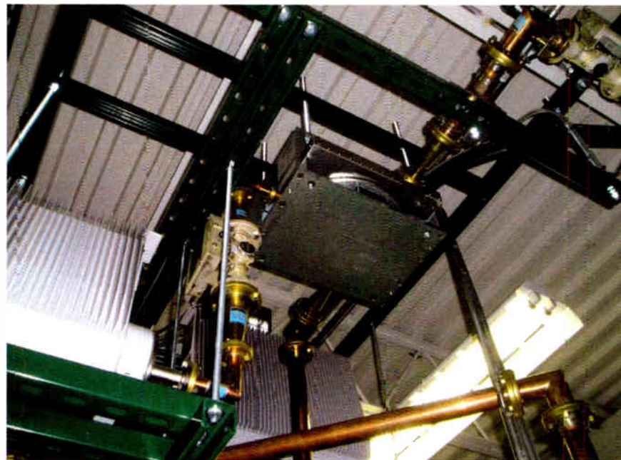
Fig. 9: Circulator installed in an FM broadcast facility.
