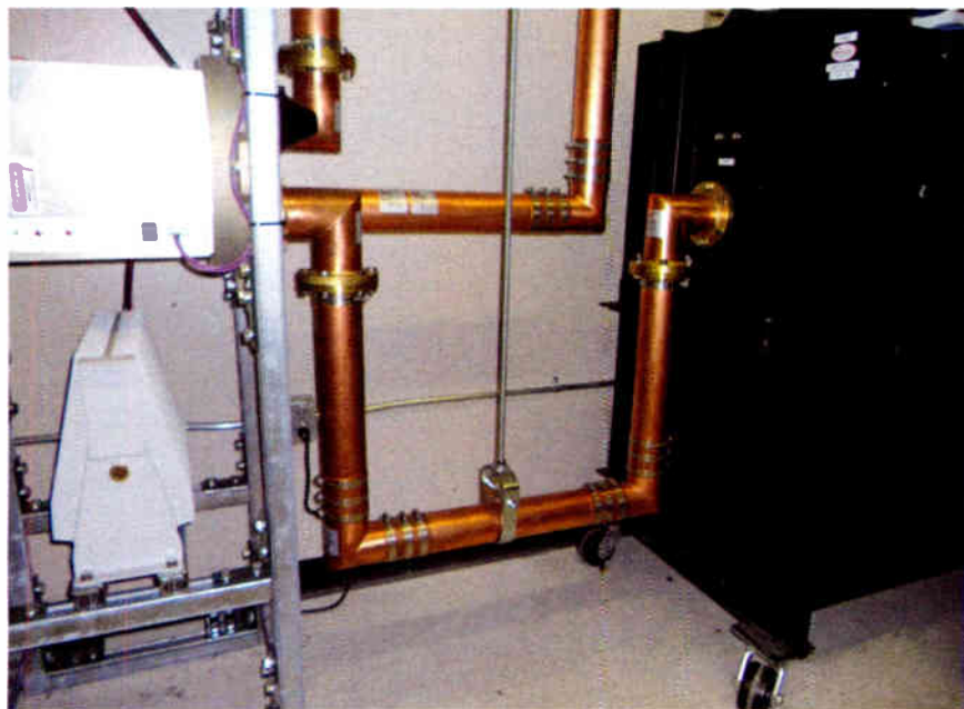
Fig. 8: 'Trombone' line ahead of a bandpass filter.
