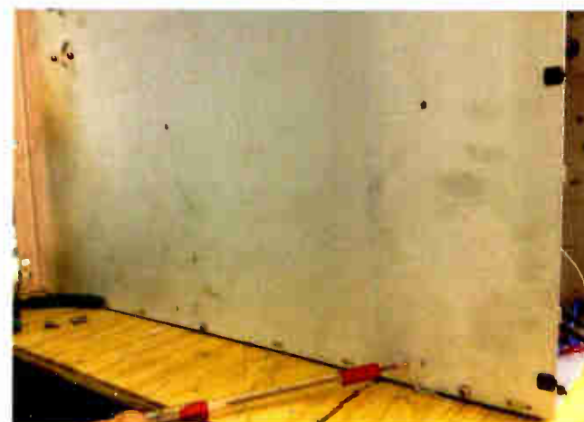
Fig. 2: Drilling holes in the side of the transmitter to mount the new supply.
