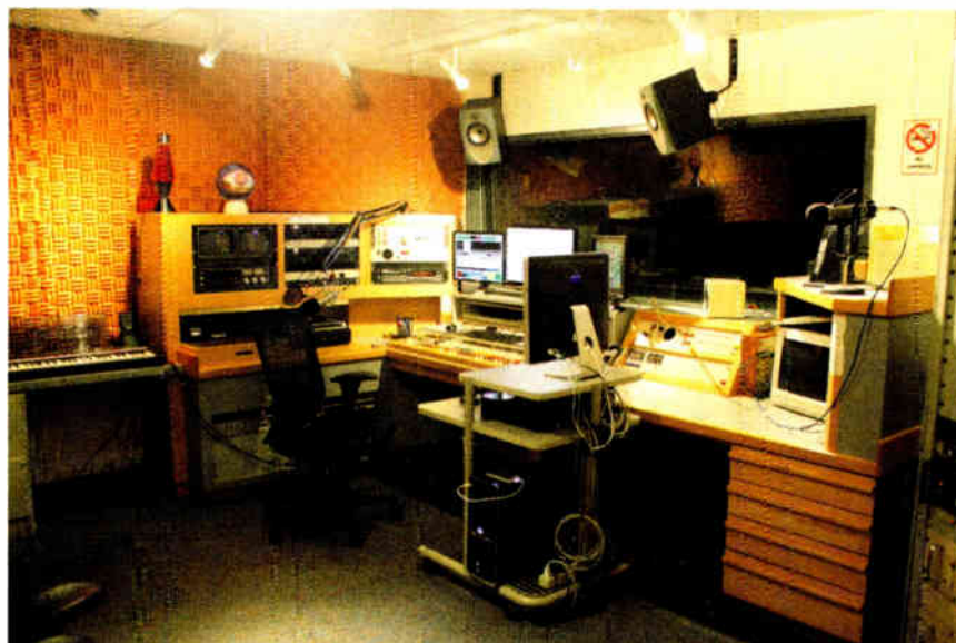
The station will move offices, news and most technical systems, including this commercial production studio, to the seventh floor of Tribune Tower. A restaurant will occupy the space.
