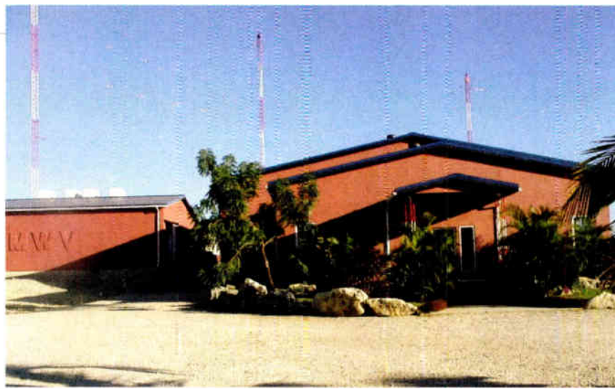
The transmitter building of the Madagascar World Voice facility, with a generator building at left. In the background are three of the four towers and MWV's three antennas.
