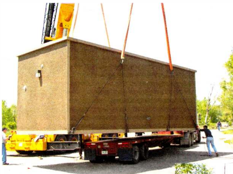
Precast shelters are shipped on 'low boy' flatbed trailers and unloaded with a crane.
