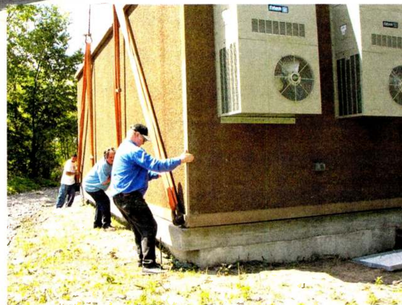
Fine-tuning the placement on the foundation slab.
