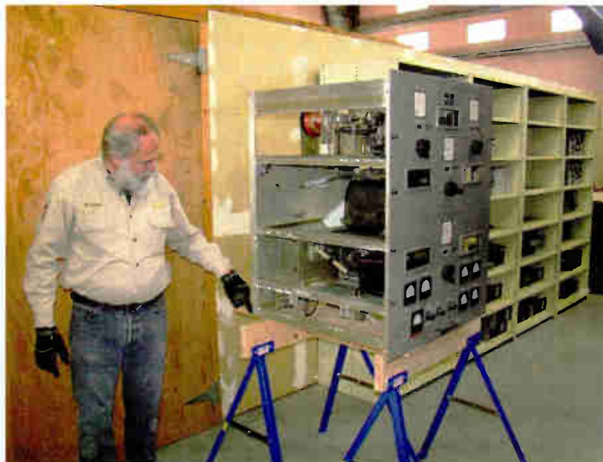
Fig. 2: The RCA T3 PA cabinet.
