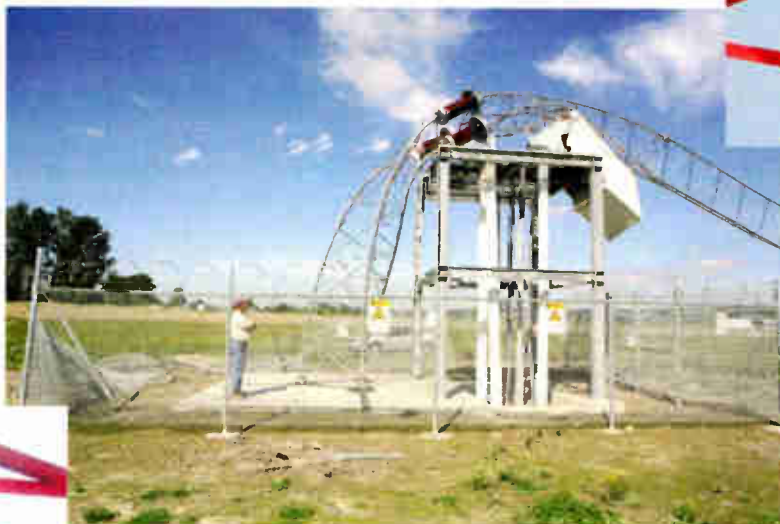
George ‘Buzz’ Anderson inspects the destroyed 199-foot antenna element and tuning units.
