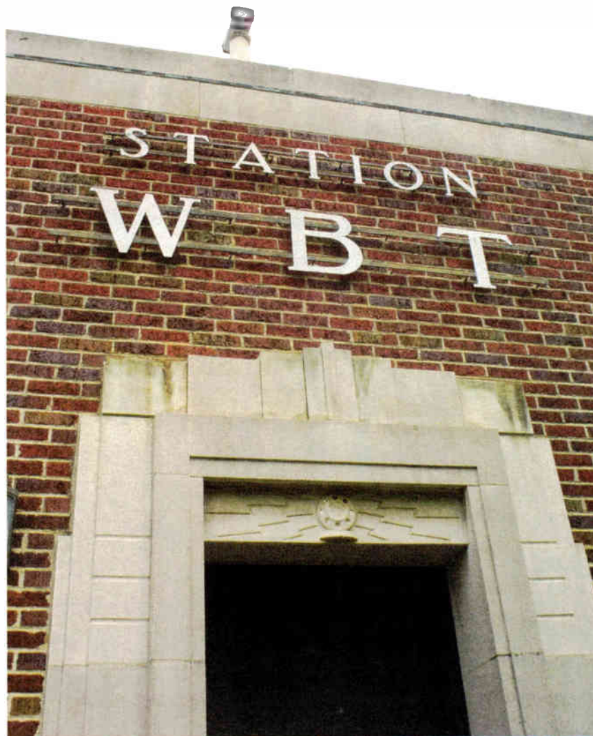
Closeup of the older building's exterior.
