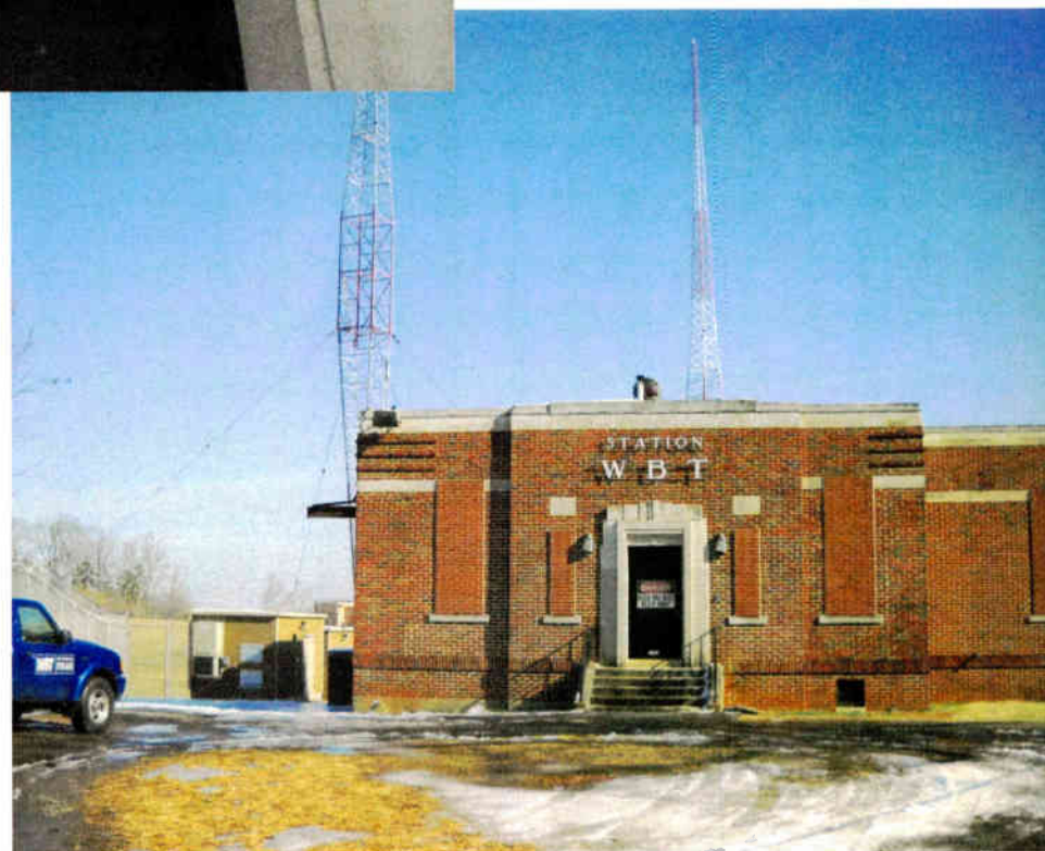
WBT's transmitter building south of Charlotte, N.C., built in 1929, houses a government underground transmission facility constructed in 1963. The new PEP station facility can be seen behind and to the left.
