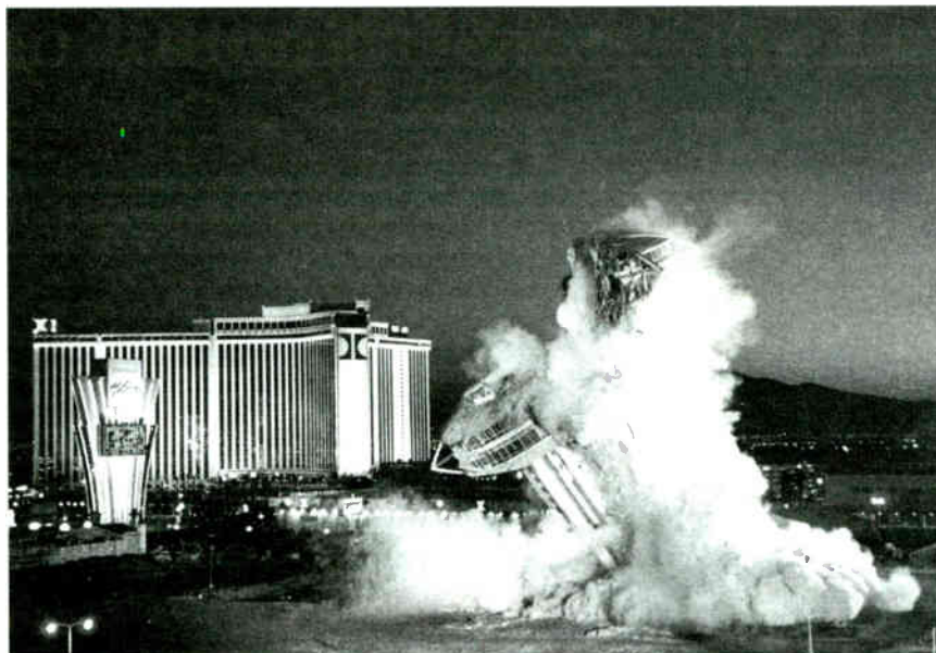
The famous Flamingo is demolished in 1995.
