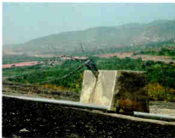
Fig. 1: Check the plumb and tension of your tower.
