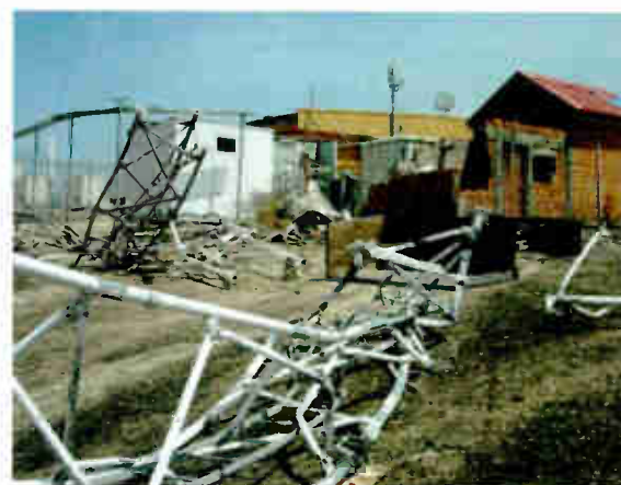
Fig. 2: A hill, high winds and a heavily loaded tower may not mix well.
