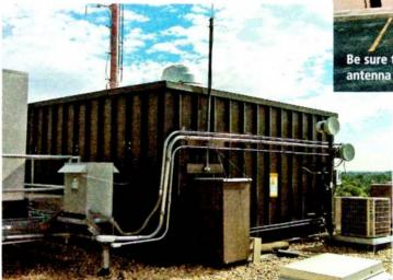
Scout the rooftop for potential STL antenna mounting locations. Parapets and elevator penthouses often make good antenna mounts.
