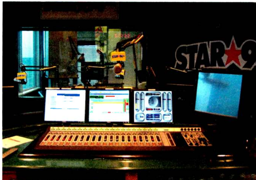
The Axia control surface atWSTR with controlling software visible on screen.
