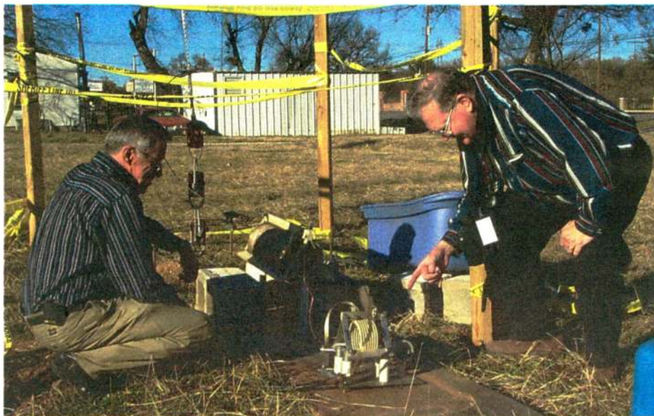
Sellmeyer, right, with Jim Jones, chief engineer of KSWA(AM) in Graham, Texas, after adjustment of the antenna coupler for an emergency 'Tee' antenna, a top-loaded vertical antenna after a tornado lopped off the upper two thirds of the tower.
