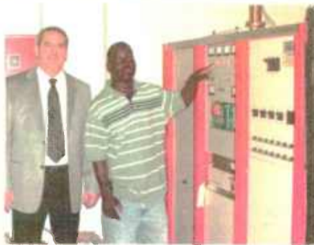
Bob Buie, left, and Andy Caston are shown at the installation of a new transmitter for WMPN(FM) in Jackson. Caston is site engineer for the station.
