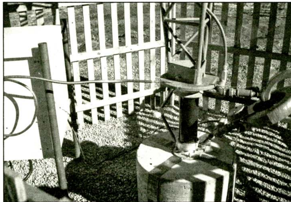
Photograph and otherwise document everything in the tower base region.
