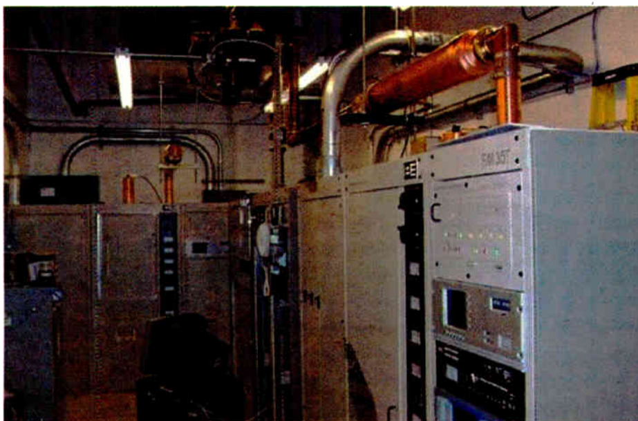
Several BE transmitters during the installation phase at WZGC.
