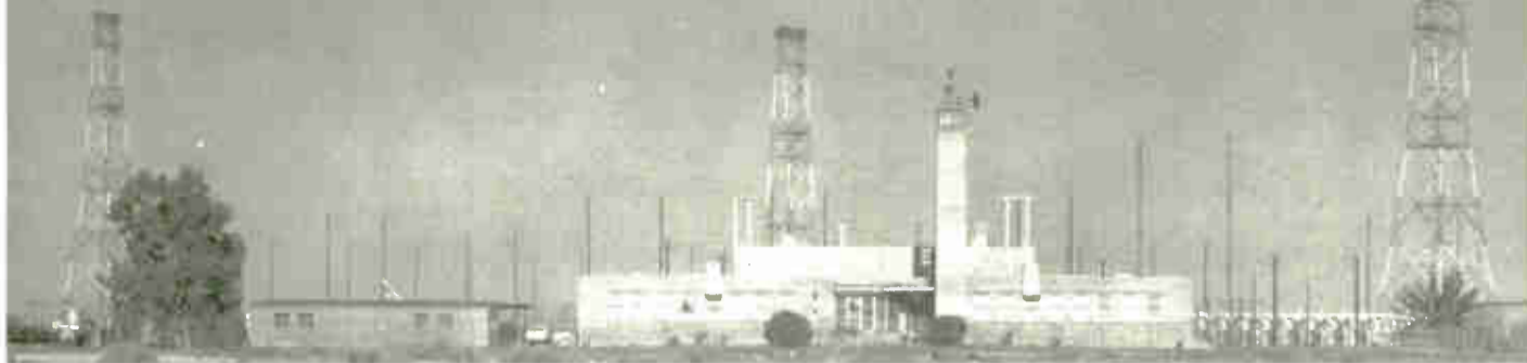
Exterior of the Delano transmitting station as it appeared in the late 1940s or early 1950s.
