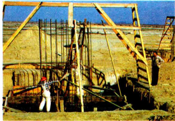
Workers prepare to pour the concrete tower base for the first of the postwar 'curtain' antennas to be installed. This is in the late 1940s.
