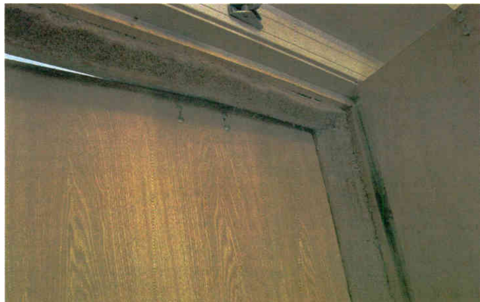
Fig. 2: A carpet strip helps deaden hall noise in this simple sound lock.
