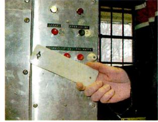
Fig. 1: Harry Bingaman used parts from his junk box to make this protective switch cover.
