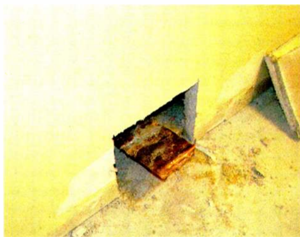
Fig. 2: Access for connecting a new pigtail
