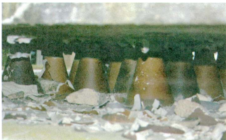
Fessenden's towers used an array of smaller insulators, rather than the large style now found at AM sites.
