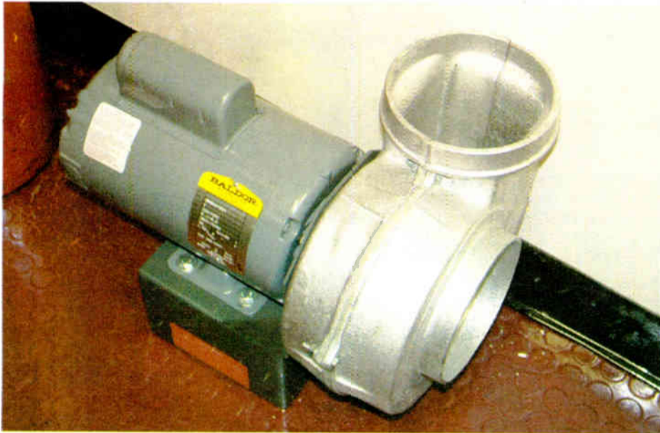
Fig. 1: Keep a spare blower motor on hand for that inevitable failure.
